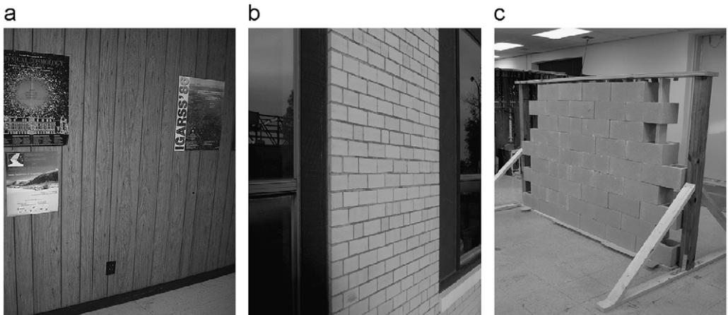
Fig. 10. (a) 5 in wooden/gypsum interior wall, (b) 15 in brick exterior wall, (c) 30 cm cinder block wall.
